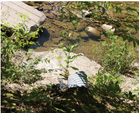
Stormwater outfalls
