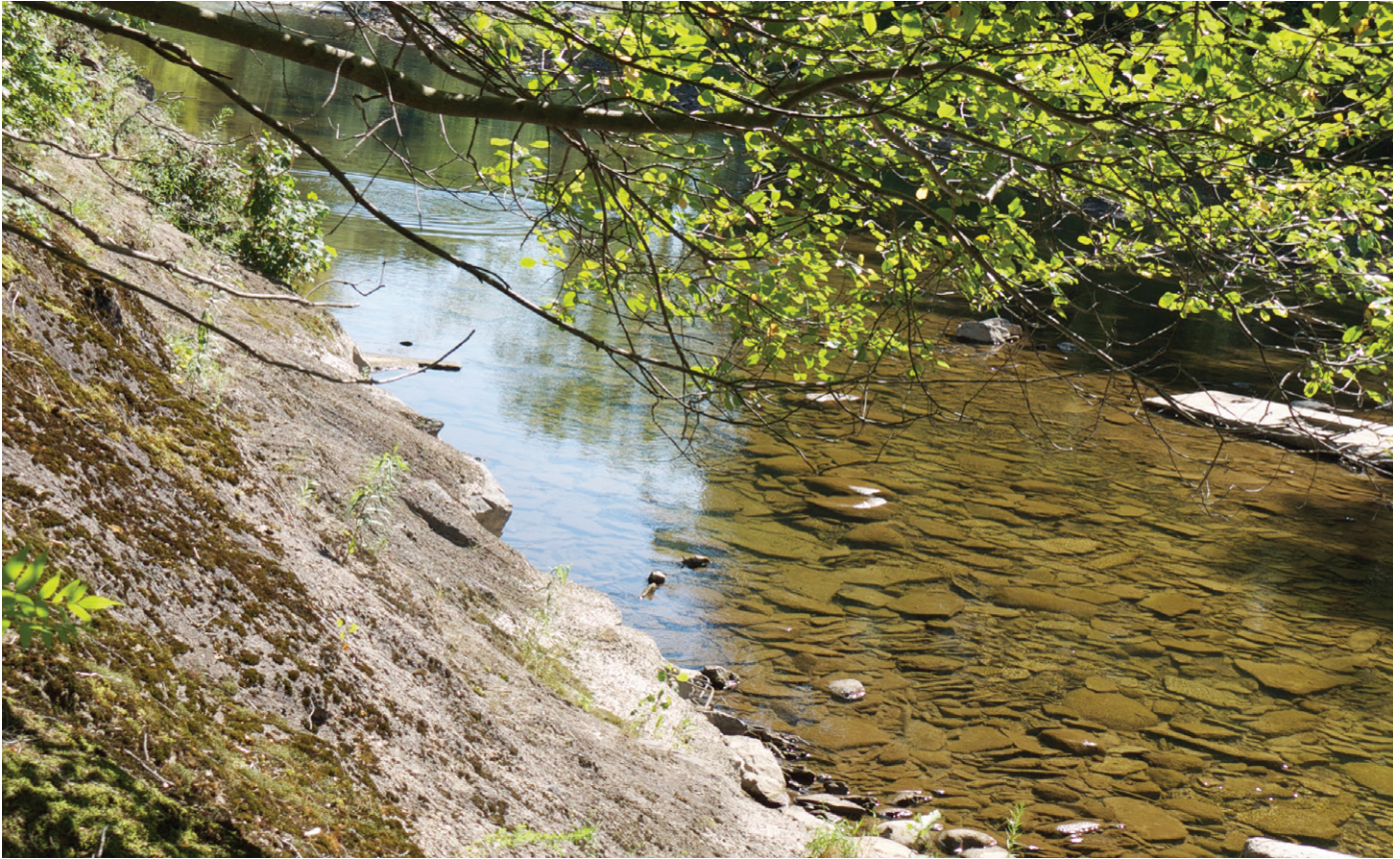
Poured Concrete Erosion Control Wall
